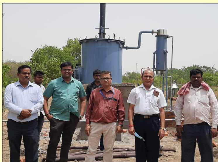
Fig. 1: Fig: Installation of Grass Oil Distillation Unit
